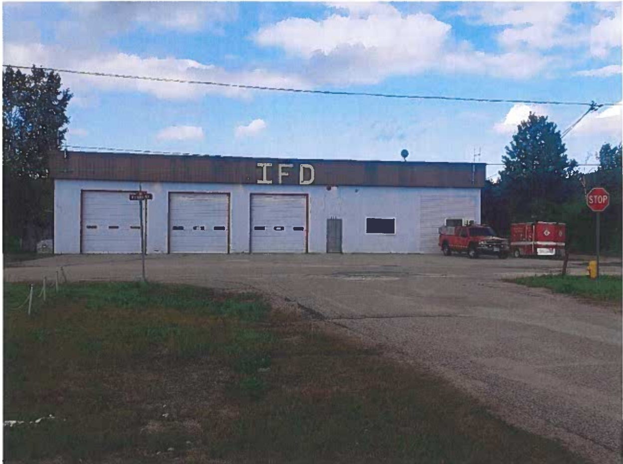
Ignace Fire Department Hall
