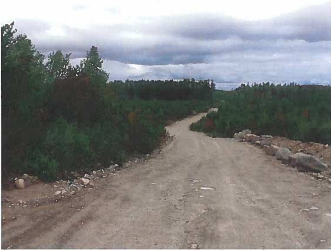
Agimak Road near the southern end of proposed fuel break
