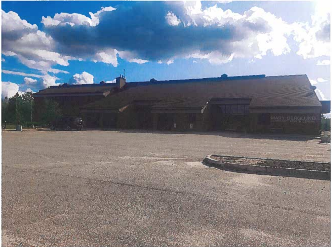
Mary Berglund Community Health Center and Service Ontario Center
