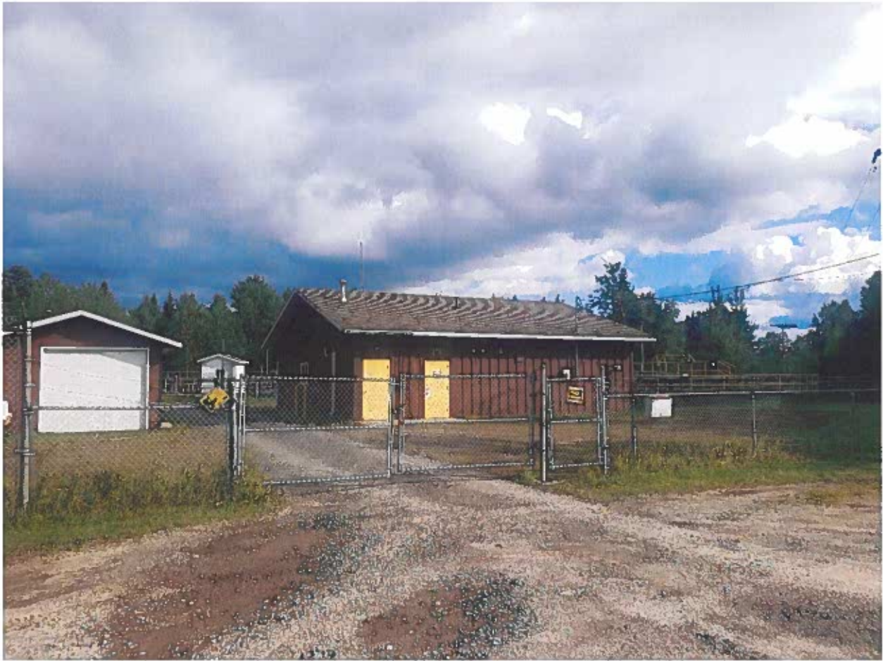
Sewage Treatment Plant
