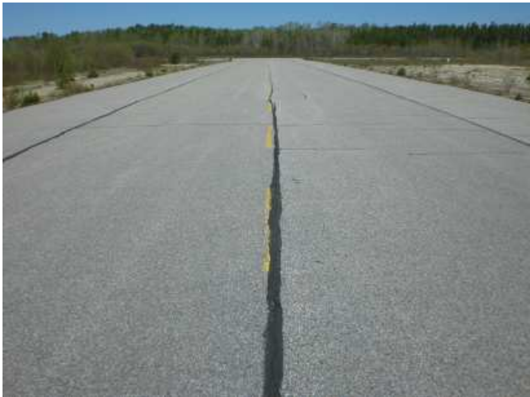
Photo No. 4 Taxiway - Longitudinal cracking (sealed)
