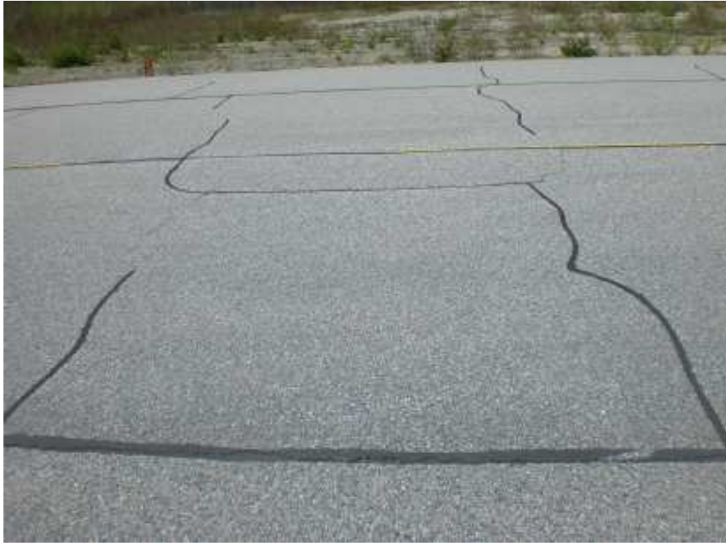
Photo No. 5 Taxiway – Typical surface defects, (sealed block cracks)
