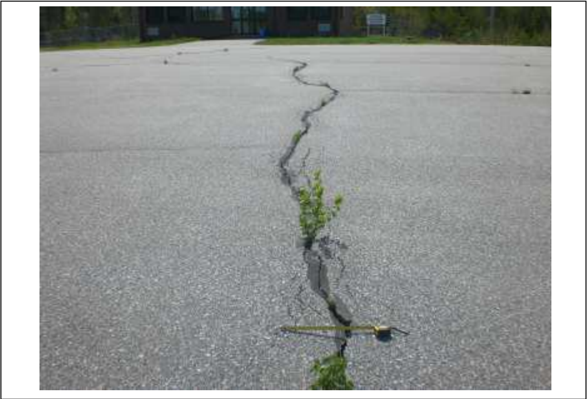
Photo No. 7 Apron – Transverse cracking. (severe)
