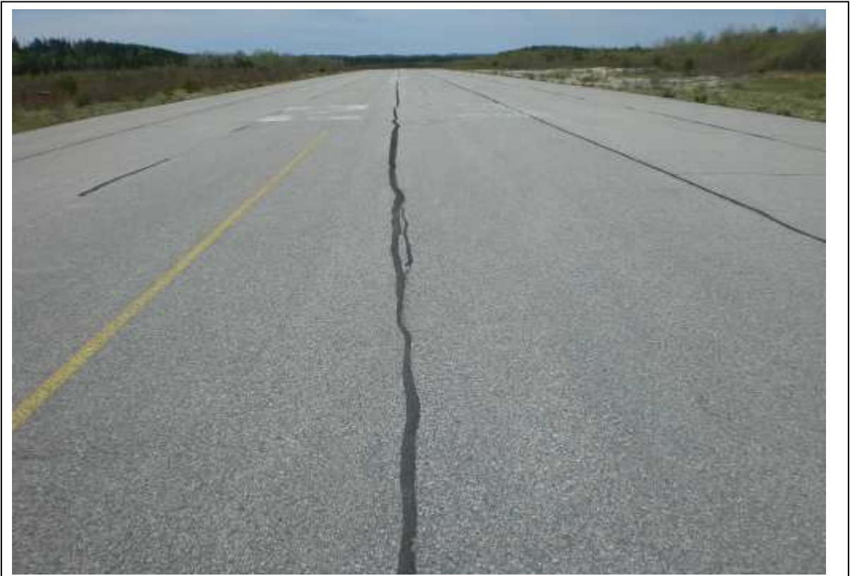
Photo No. 1 Runway 05-23 – Longitudinal cracking (sealed)
