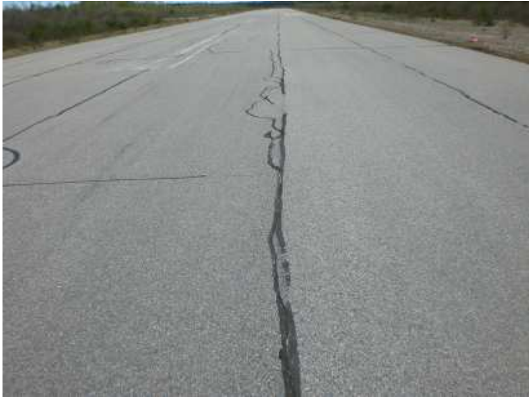
Photo No. 3 Runway 05-23 – Typical surface defects
