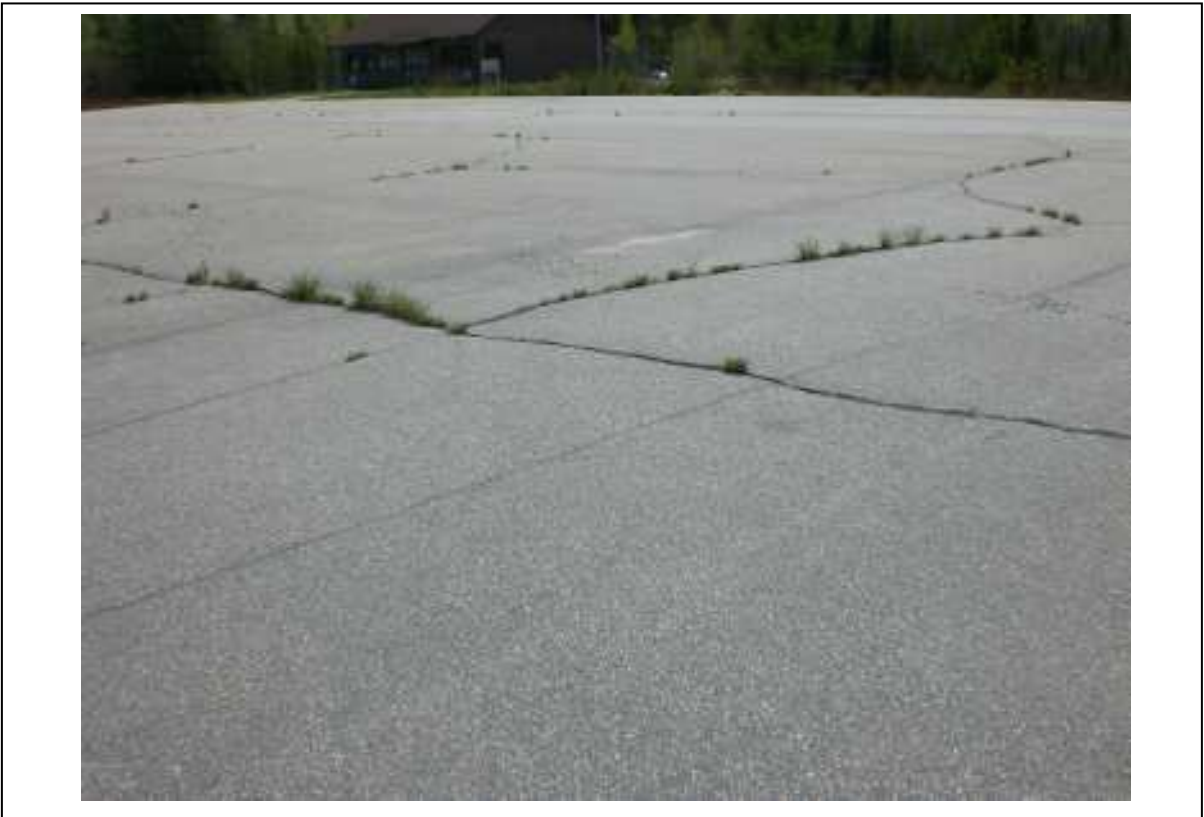
Photo No. 8 Apron – Typical surface defects.
