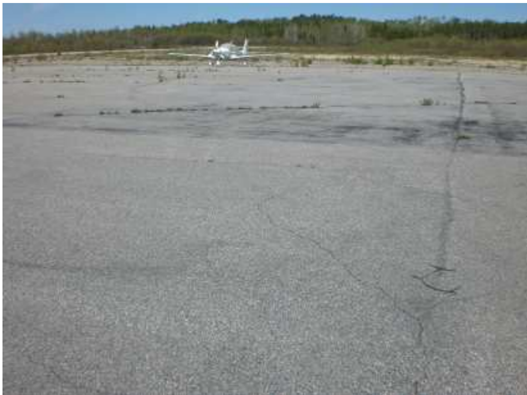
Photo No. 6 Apron – General View
