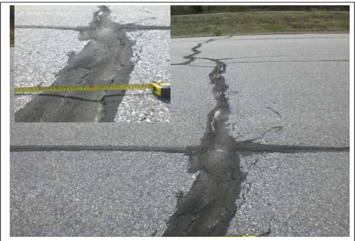
Photo No. 2 Runway 05-23- Severe transverse cracking (sealed) with subgrade settlement.
