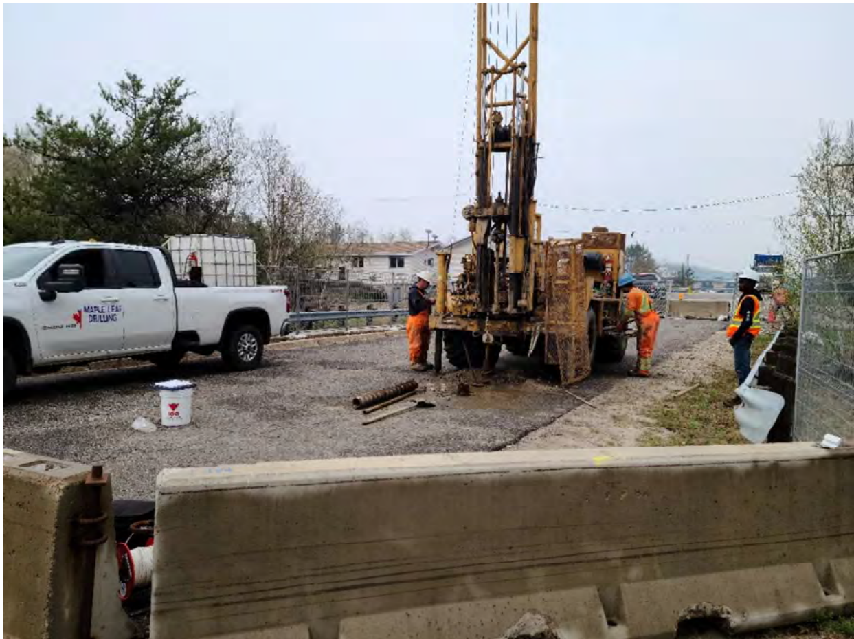
Photo 2: Completion of Borehole 2 drilling at Pine Street Culvert.
